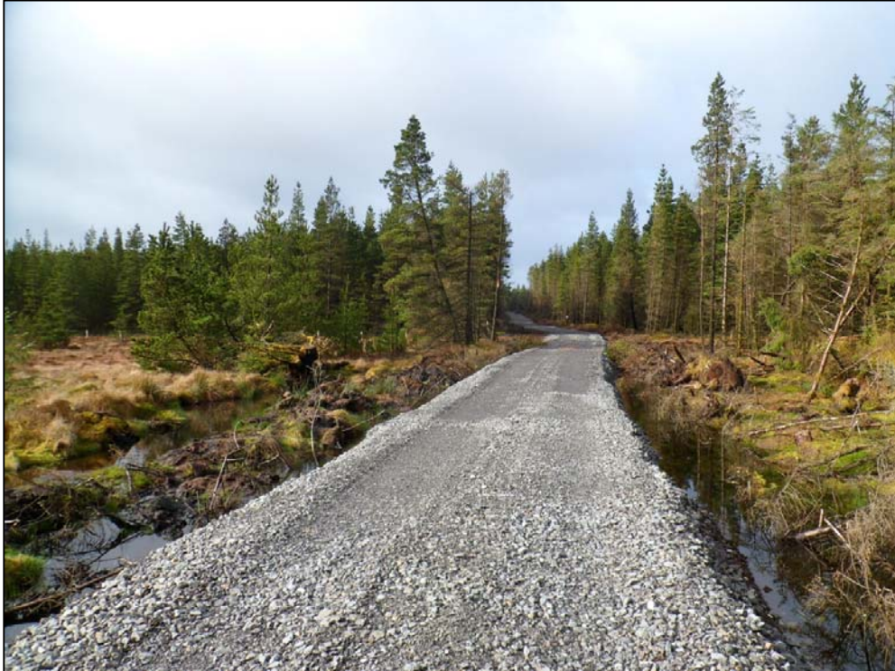
Photo 7 Example of floated access track on site
