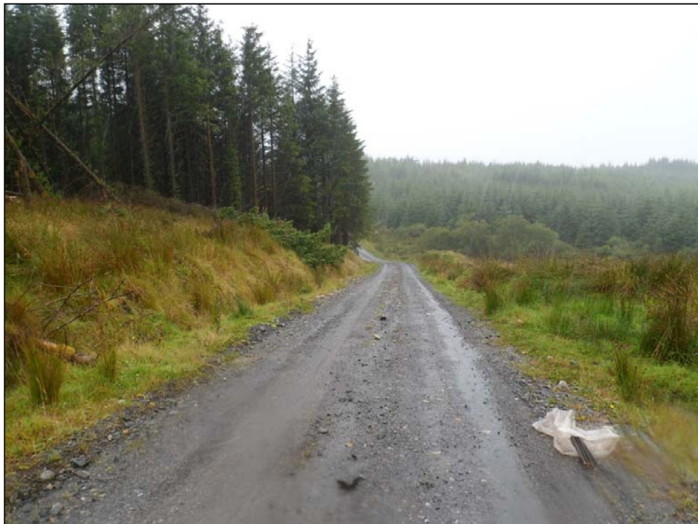
Photo 6 Example of founded access track on site
